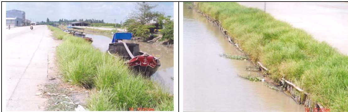
Photo 8 Vetiver dike protection
